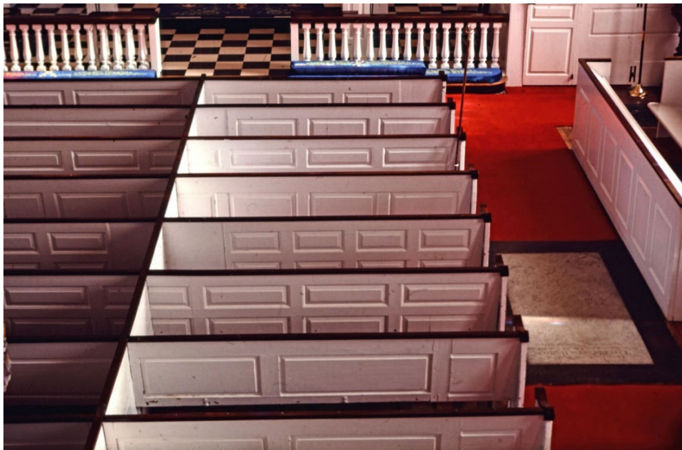
Detail showing the paneled square and long pew parts as reconfigured in 1844 into slip pews of uniform length. Author's image.
