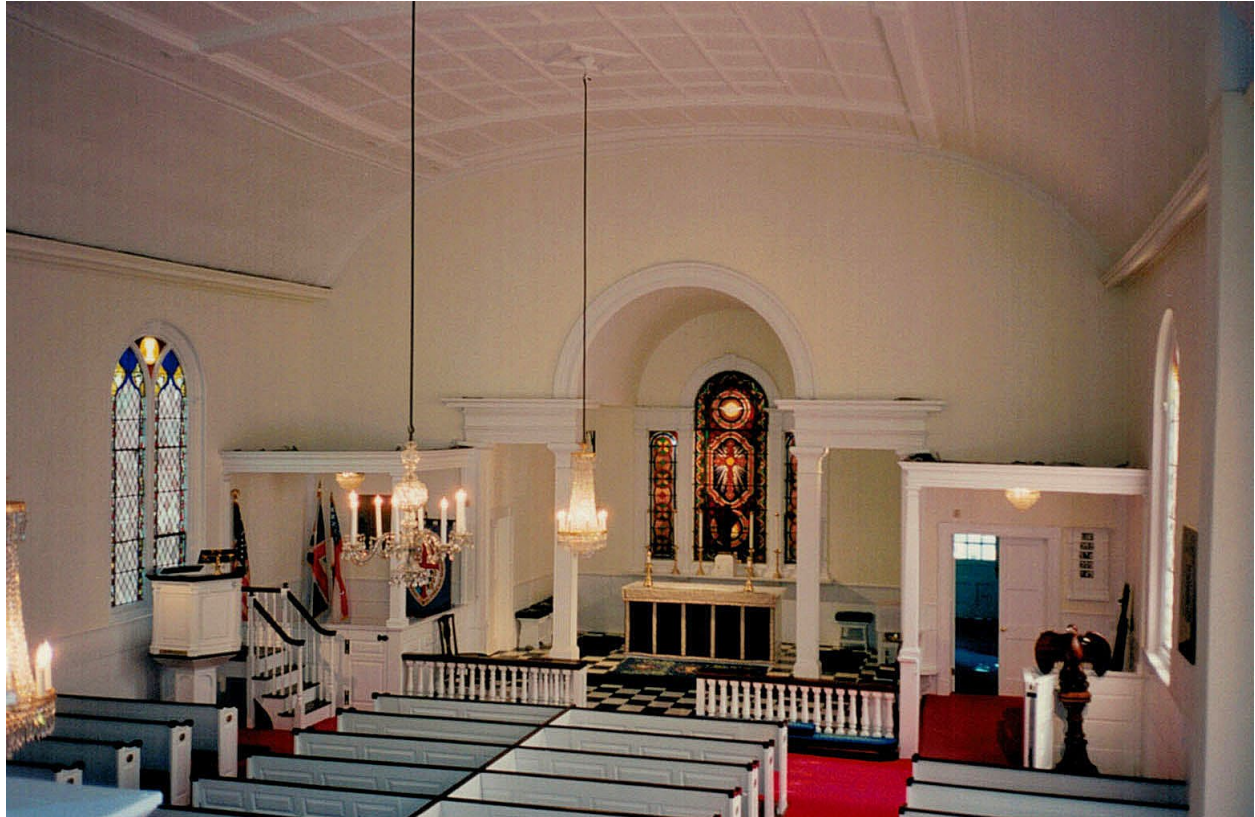
The interior of Christ Church, Shrewsbury as it appears today. The two original canopied pews flank the 1844 chancel recess. The raised bottom chord roof trusses allowed for the graceful arched ceiling which is now ornamented with pressed tin installed in 1906. Author's image.
