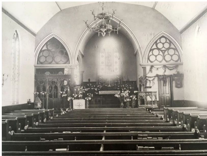
The interior of St. Peter's Church, Freehold, as it appeared between 1892 and 1896. The high arched ceiling, restored in 1878, follows the profile of the original ceiling. Courtesy St. Peter's Church.
