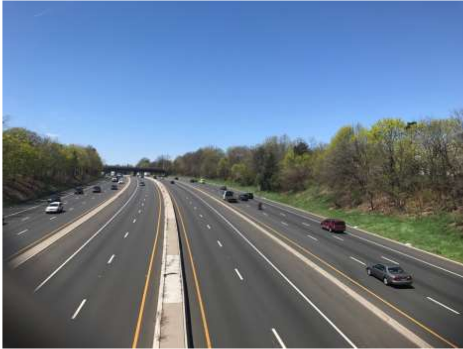
Photo taken by author, April 15, 2017, from Osborne Terrace Bridge spanning Route 78 facing west.
