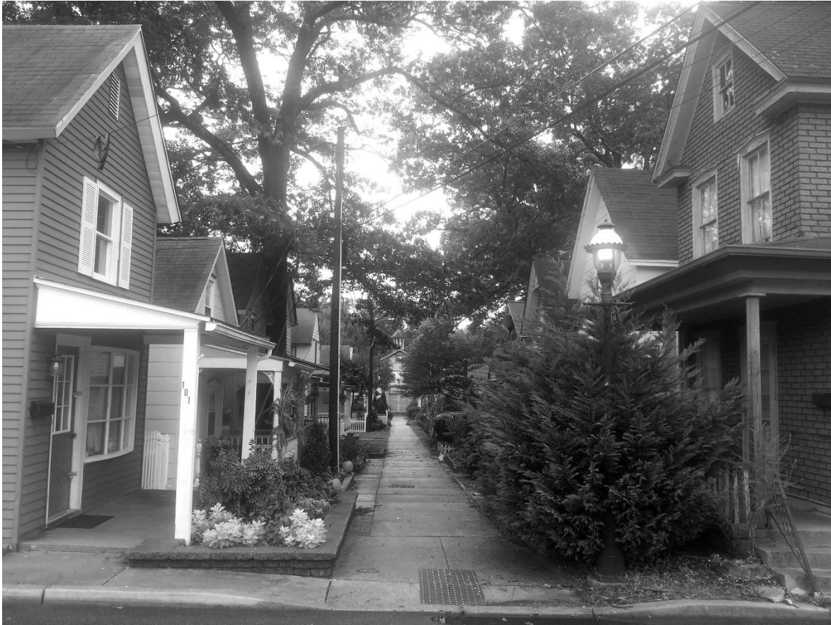
Cottages lining First Avenue, with the recently remodeled Pitman Grove Auditorium in the distance. 173
