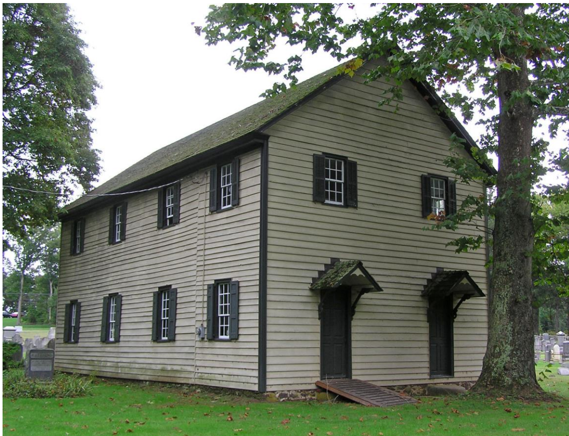
A view of the meeting house from the northwest, showing the 1836 extension and its two entrances. A vertical line in the siding to the left of the electrical service marks the joint with the earlier part of the structure.
