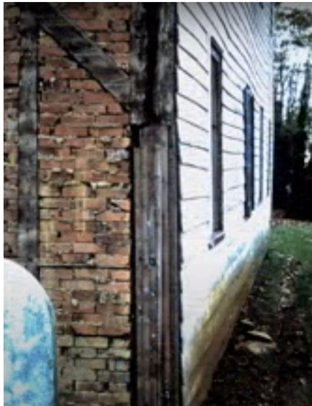
An old repair of the northeast corner post exposed in 1977/78, pieced out roughly six feet. Courtesy OYMH Slide Show.
