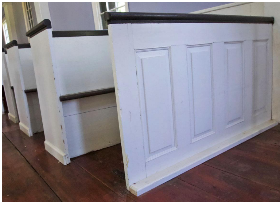
Detail of a paneled pew frontal and simple board pews on the first floor of the meeting house. The paneling matches similar woodwork on the sides of the pulpit platform and west gallery stairs. Courtesy Sheila Koehler.
