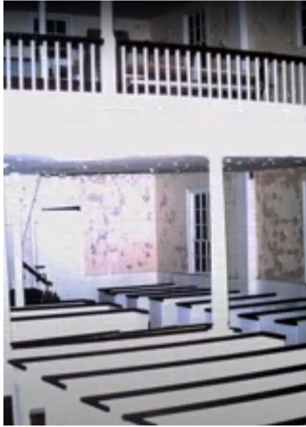
The west end of the meeting house interior before rehabilitation. Note the deteriorated condition of the paint finishes on the plaster walls and ceiling under the gallery, which had peeled extensively. OYMH Slide Show.
