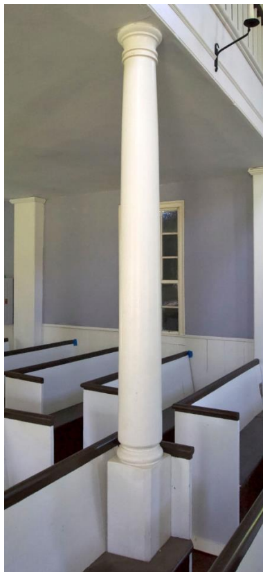
Detail of an attenuated turned column that supports the west gallery. Courtesy Sheila Koehler.
