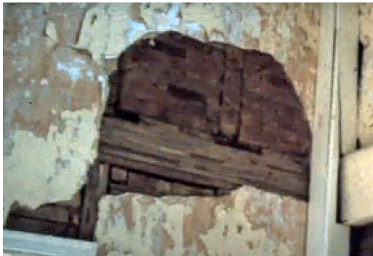
A cut off support timber for the east gallery was uncovered during restoration work in 1977/78. It can be seen sitting on the top surface of the exposed wall girt where plaster had been removed. Note also the pale yellow paint on the plaster, with light blue showing under it. Courtesy OYMH Slide Show.
