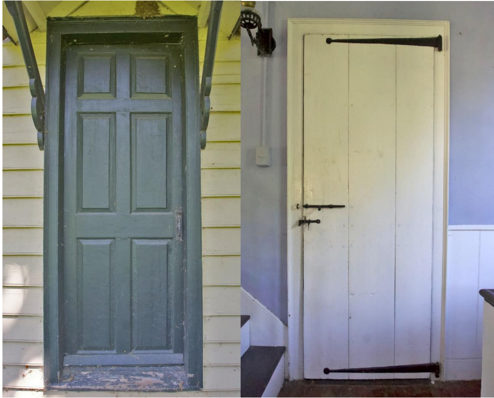
Exterior and interior views of the north door on the west elevation. Note the early wrought iron strap hinges, as well as the iron latch and lock. The exterior hood over the doorway was added in 1877. Courtesy Sheila Koehler.
