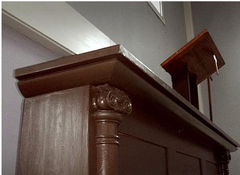
Detail of a carved Ionic capital, column, bold moldings, and flat panels that ornament the 1836 restrained Greek Revival pulpit, which is made of cherry wood. The reading stand is a recent addition. Courtesy Richard Lore.
