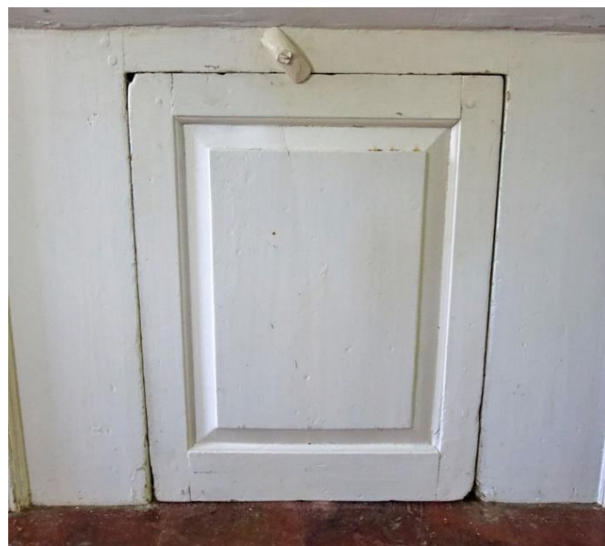
Detail of the small piece of eighteenth-century paneling reused as an access panel under the gallery stairs. Courtesy Sheila Koehler.
