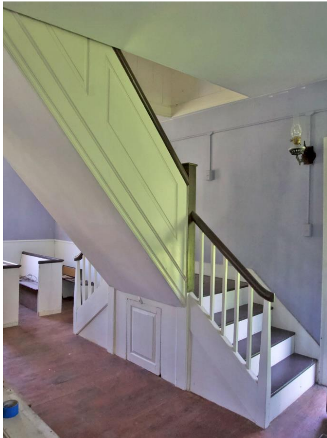
The unusual T-shaped stairway to the west gallery featured raised paneling. Courtesy Sheila Koehler.
