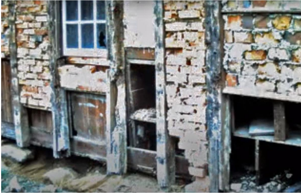
Severe deterioration of the sills, wall studs and brick nogging was discovered in the south corner of the east elevation in 1977/78. The back of the raised pulpit platform can be seen on the right. Courtesy OYMH Slide Show.
