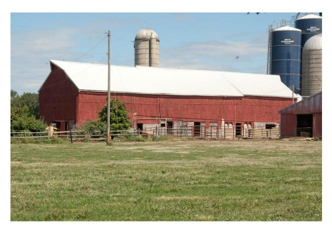
Figure 4. The Bassett-Allen-Waldac Farm, Mannington Township, features a dairy barn composed of three, four-bay threshing barns. The first one (situated in the middle) is dated 1792 and is flanked by two others built before 1848 and before circa 1860. They were strung together and widened for expanded diarying and fodder storage. The loft was also used for ballroom dances. Photo by the author.
