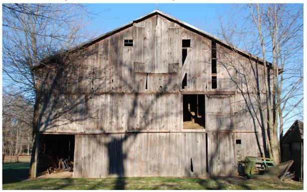
Figure 6. Henry and Elizabeth Freas farm, Alloway Township. This 1895 barn replaced one destroyed by fire. This gable-fronted barn has four bays accessed via sliding doors. Left to right: a wagon drive-through, a feeding aisle, a milking aisle with wood stalls, and an open forebay on posts. Hay mows above. Photo by the author.
