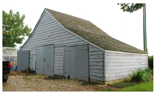
Figure 8. Caspar & Rebecca Wistar Wagon House illustrating the broken roof slope type which accrued over time. This one began as a pentagonal or keystone-shaped drive-through corn crib. Shed additions were later attached, first below the main eaves, then raised to meet the upper roof slope. Here, there is no cellar or loft. Photo by the author.
