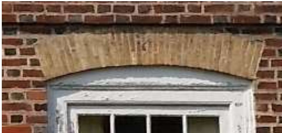
Rubbed and gauged bricks formed into a relieving arch. William Trent house detail. Photograph by the author.
