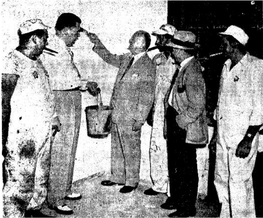
Leo J. Rodgers Homes construction site featured in Trenton Evening Times ; second to the left is Joseph S. Tysowski, Director of Tenant Relation for the THA. Trenton Evening Times , July 28, 1948.
