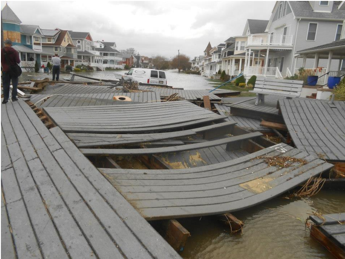
Tossed boardwalk and swamped van at Ocean Avenue and 8th Avenue, Belmar. Photograph courtesy of Monmouth County resident Jenna Amore Wheeler.
