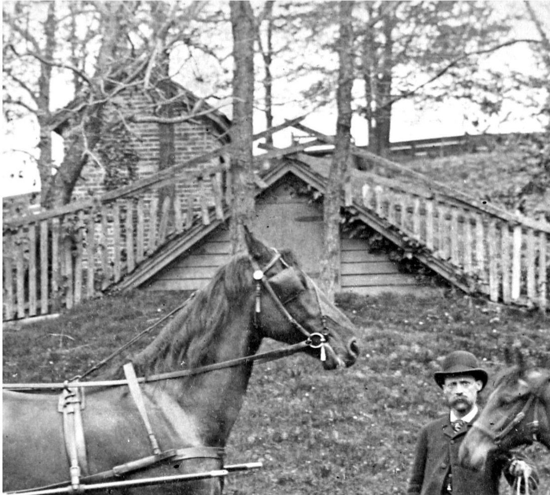
Detail from a larger photograph which shows the ice house and smoke house at Orchard Home, taken about 1890. Although in severely deteriorated condition, the smoke house still stands. Note the unusual manner in which the picket fence along the driveway goes over the gable end of the ice house. Edward Taylor photograph. Taylor Family Papers.
