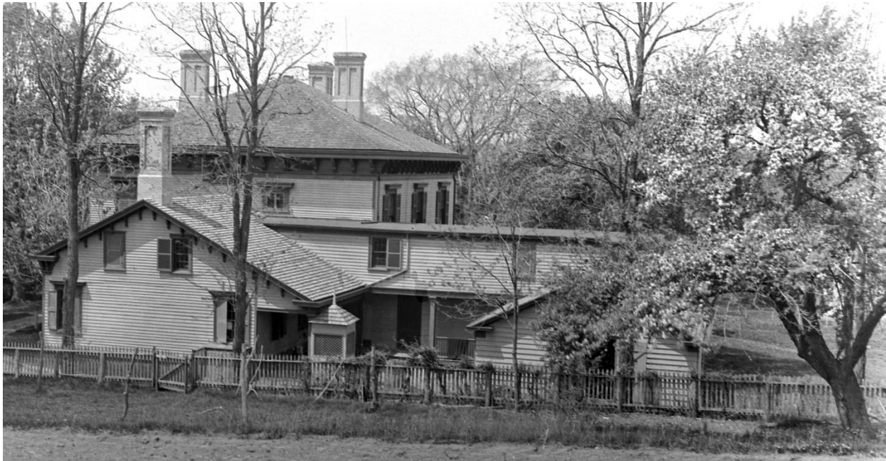
Orchard Home as seen from the kitchen garden, taken about 1890. The service courtyard is shown with the single story kitchen wing to its left and a storage shed on its right, with the bridge from the main residence to the two story privy passing overhead. Edward Taylor photograph. Taylor Family Papers.
