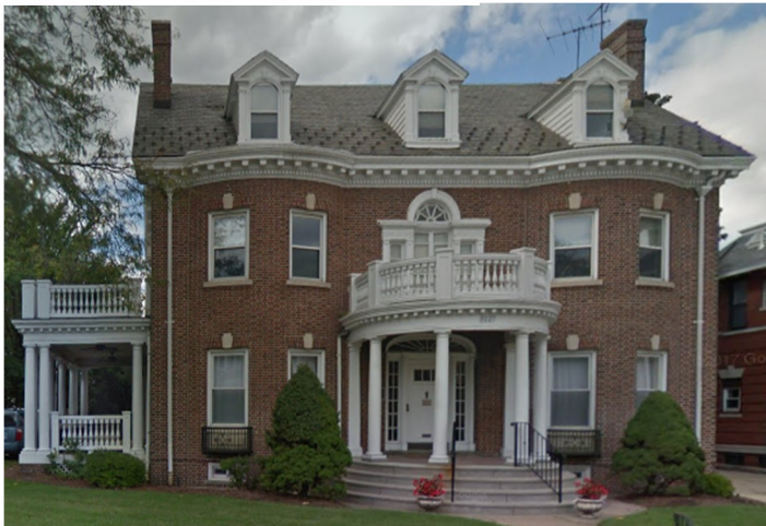
2627 Kennedy Boulevard (Google Street View)
