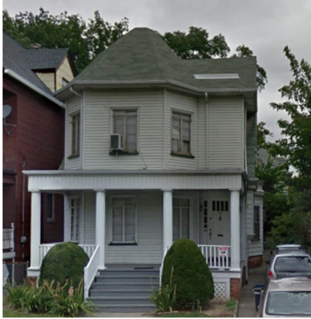
242 Harrison Avenue (Google Street View)
